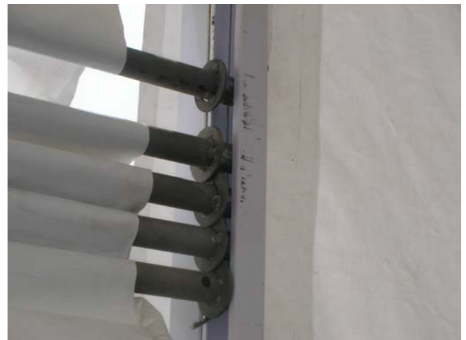
Door Tubes Inserted Into Door Track
