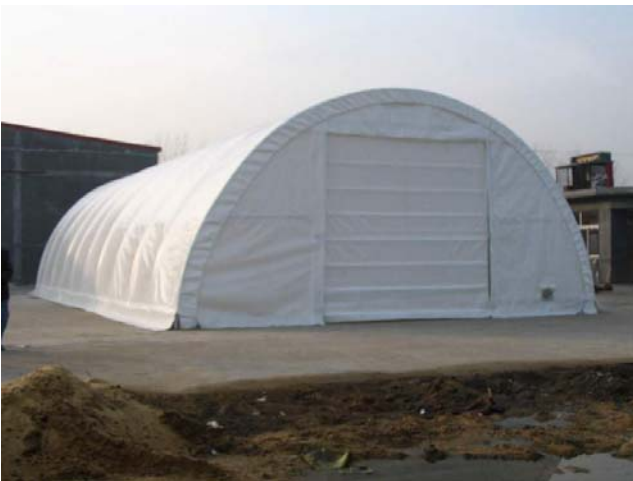
Building Completed Main Roll Up Door in fully Open Position
