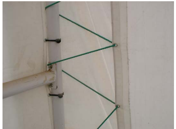
Rope Lacing Main Cover Front-Back
