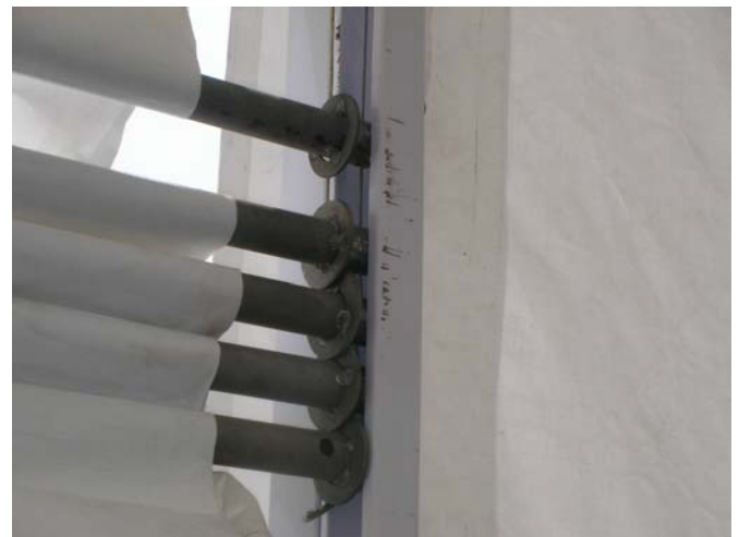
Door Tubes Inserted Into Door Track
